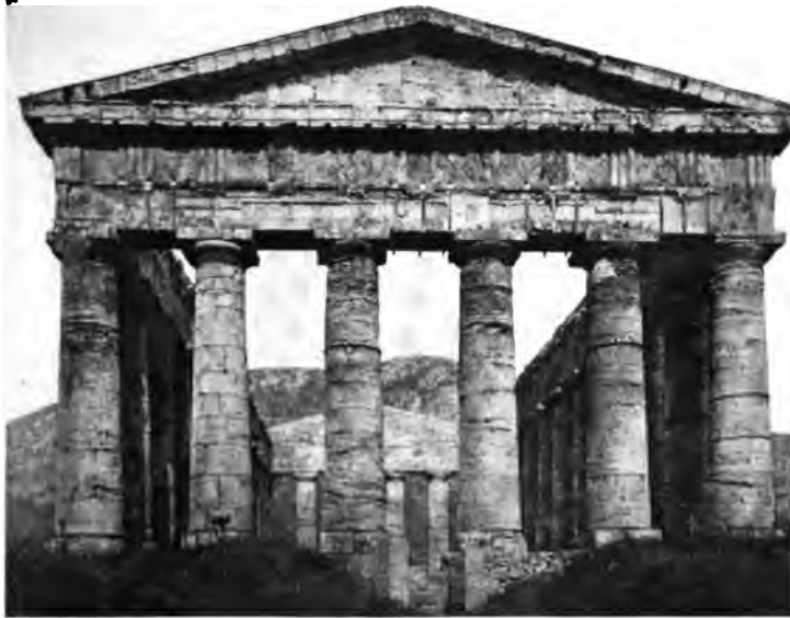
AN EARLY EXAMPLE OF THE GREEK DORIC TEMPLE (UNFINISHED) The columns here are heavy and spaced closely together. The flutings of the columns, as well as mouldings of pediment and cornice, would have been carved "in place," had the work been completed (Temple at Segesta, Sicily)
